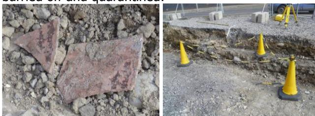
A sample was taken, double bagged and sealed before being taken to be analysed. The result of the sample was received within 24 hours. The sample has been confirmed as chrysotile asbestos. The principal contractor is arranging for a licensed contractor to remove all of the material and to dispose of it as hazardous waste. When excavation in an environment which has been industrialised for many years always be aware that asbestos, in some form or other, may have been buried indiscriminately.
