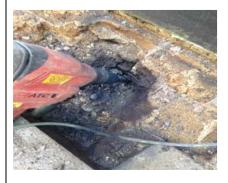
A recent incident (non-VGC) incident involving a cable strike resulted in serious electrical burns injuries to the operative undertaking the groundbreaking activities.
