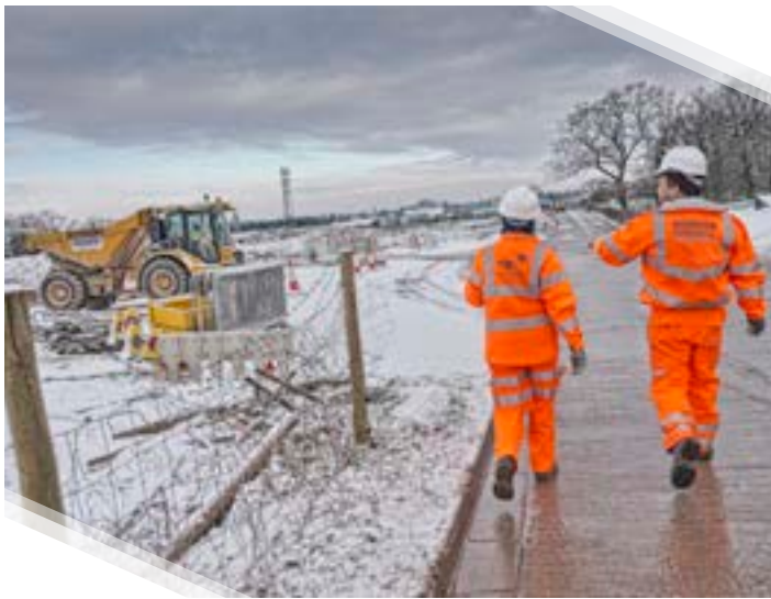
Works on the A6 Manchester Airport Relief Road
