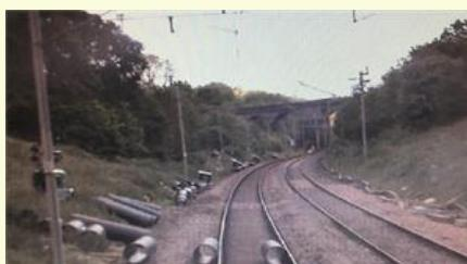
The pipes had been left on the lineside by contractors doing drainage work in the area during available possessions. The pipes had not been secured against vandals. An investigation will explore whether they were moved by vandals or by the physical effects of passing trains.
