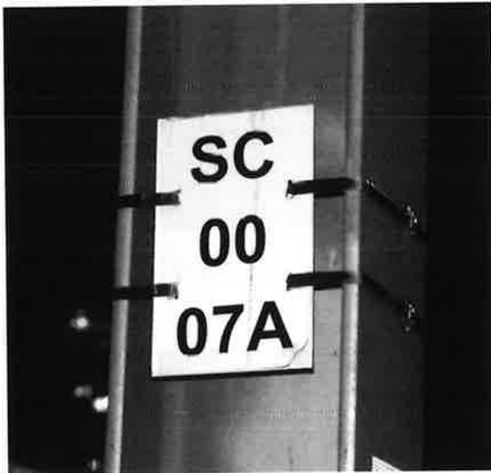
An OLE structure plate, which will identify where you are to a ECO.
